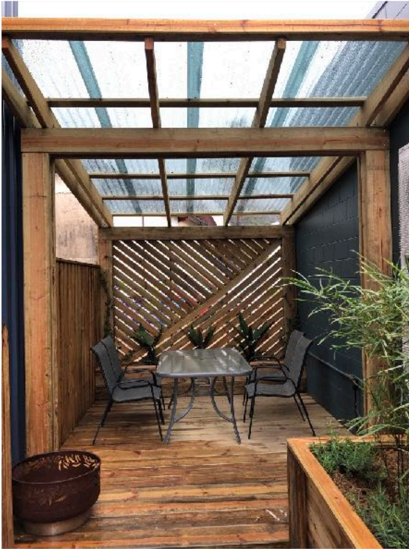
SLEEPER & FENCE RAIL PERGOLA POSTS AND BEAMS
